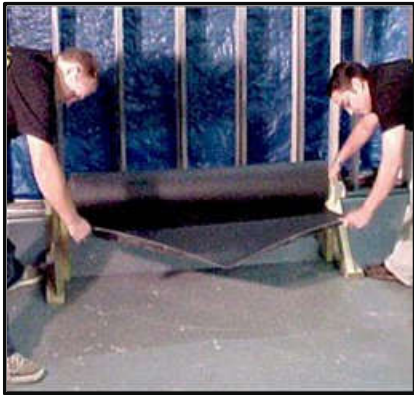
Place the roll of BlastBlock on the floor, then cut to length
